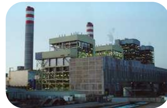
Jorf Lasfar thermal plant
